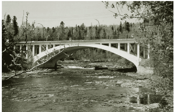
The Black Bay Bridge in the City of Thunder Bay is one of the first single span, reinforced concrete bridges ever constructed. Constructed in 1912, this singular span bridge was designed to harmonize with the beauty and grandeur of the landscape. (Photo: Ministry of Culture)
