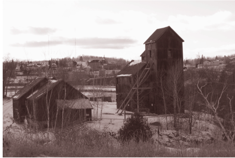
Townsite Shaft 1 Headframe, Cobalt (Photo: Ministry of Culture)
